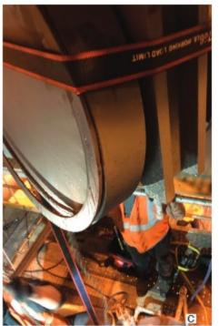
1. Removal of damaged seats and reinstallation of new ones is a job for experts capable of quality work in uncomfortable positions (A). Examples of seat (B) and disk (C) delamination illustrate typical damage to these critical valve parts. Stellite overlay has been welded on new disc (D) with an Inconel butter layer between the F91 base material and hardfacing. Final machining of the stellite overlay on valve seat is in progress in (E), finished
